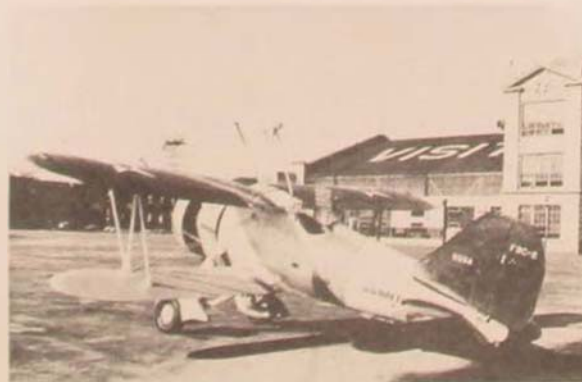
U.S. experimentation with the piggy-back concept dates to the 1920s, when the Sperry Messenger, (shown above during two stages of restoration) was tested at McCook Field, Ohio. The hook on the top wing engaged a trapeze grappling apparatus hanging from an airship. . . . In the early 1930s the Navy's Sparrow Hawks (right) attached to the dirigibles USS Macon and Akron, three of them being destroyed in the Macon disaster on 12 February 1935.
